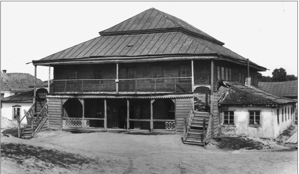
Figure 4 The Great Synagogue, exterior view from the south-west. Photo: Henryk Poddębski, 1925. Reproduced by courtesy of the Instytut Sztuki, Polish Academy of Sciences, Warsaw
