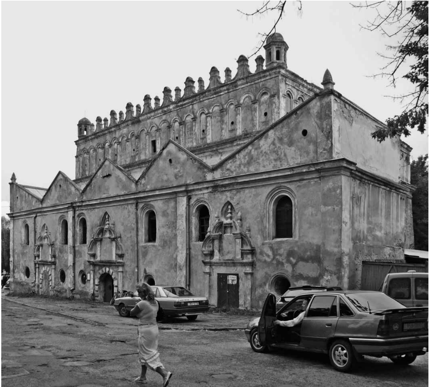
Fig. 8. The Great Synagogue of Zhovkva, 1692. View from south-west (photo: Sergey Kravtsov, 2006)
