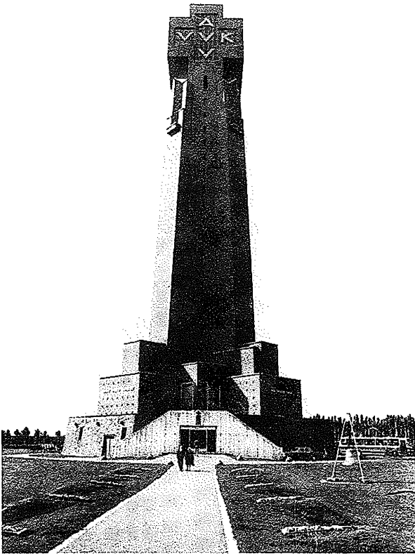
FIGURE 17.17. Tower of the Yser, Dixmunde. Razed in 1946, rebuilt after 1952.
