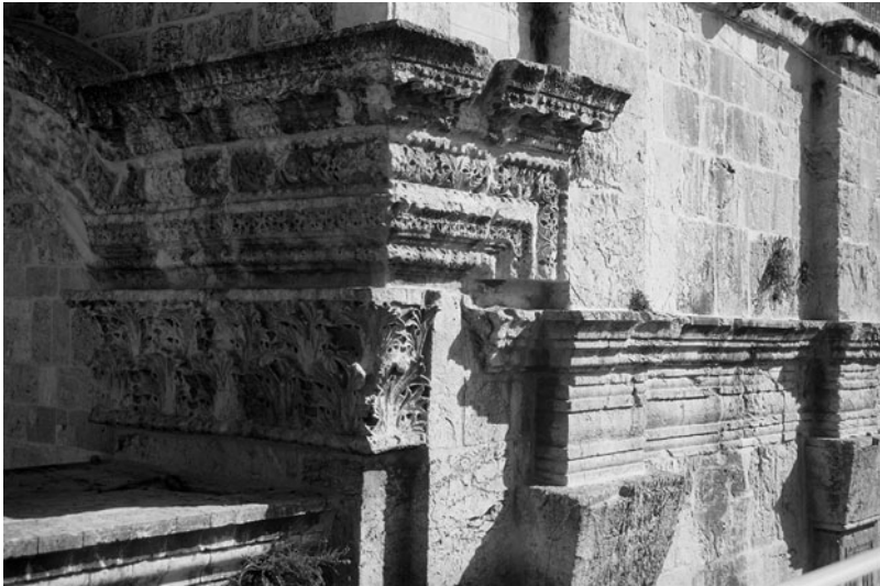
Fig. 9.4. Detailed architrave and cornice of the southwestern corner of the Golden Gate. Photo H. Bloedhorn.
