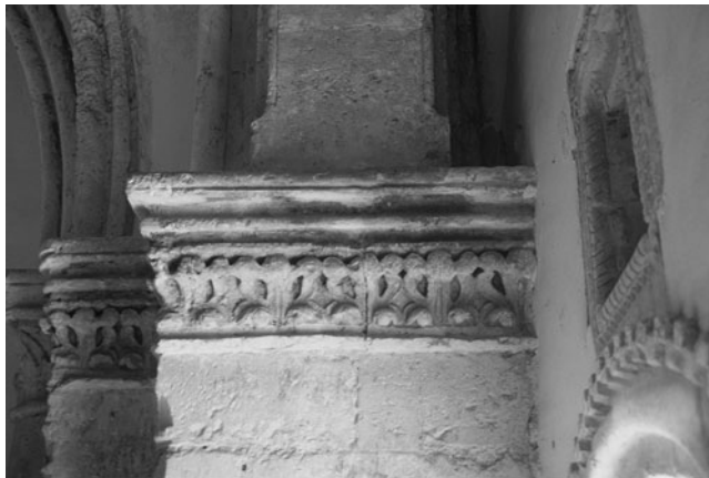
Fig. 10.14. Southern pillar with two buttresses; the right one pointing toward the nave of the former church of St. Mary on Mount Zion, the left one pointing toward the southern aisle. Photo H. Bloedhorn.
